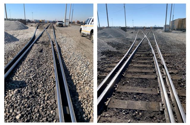
The picture on the left represents a reoccurring gage condition caused by improper alignment.
