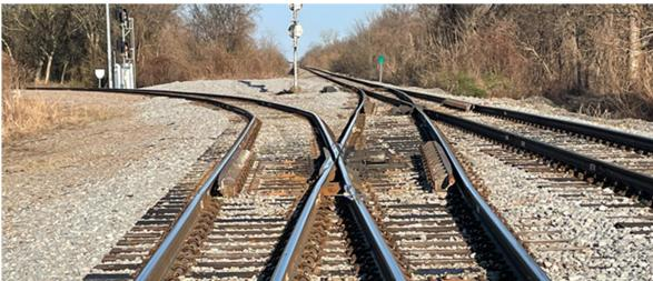
After taking the alignment measurements we originally had 12" of alignment within 31 feet, now down to under 5".
